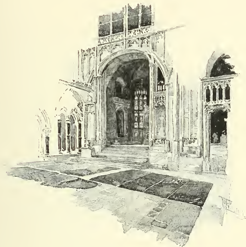
ST. PAUL'S CHAPEL, NORTH ARM OF TRANSEPT.
